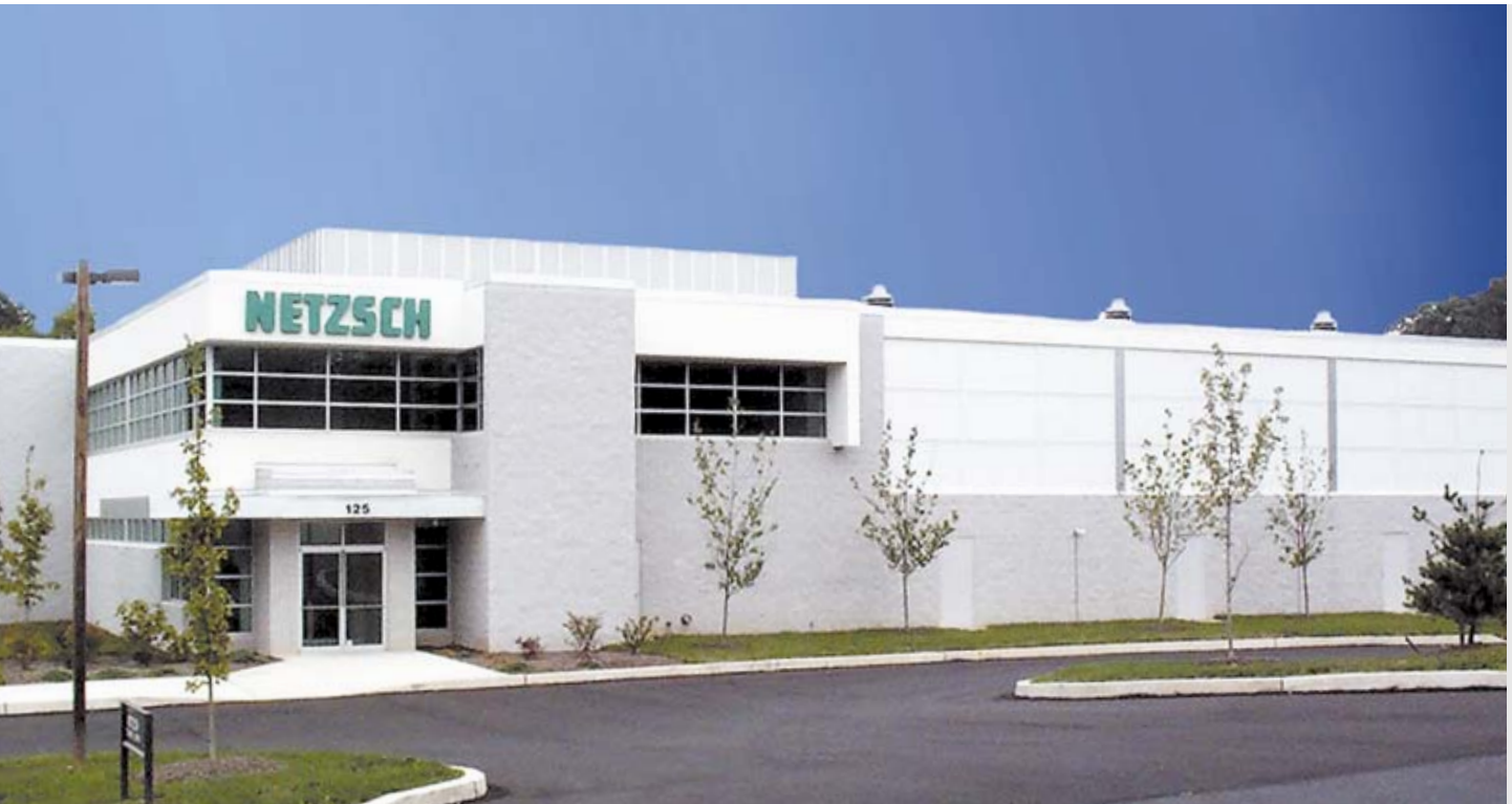
Exton, PA Facility
