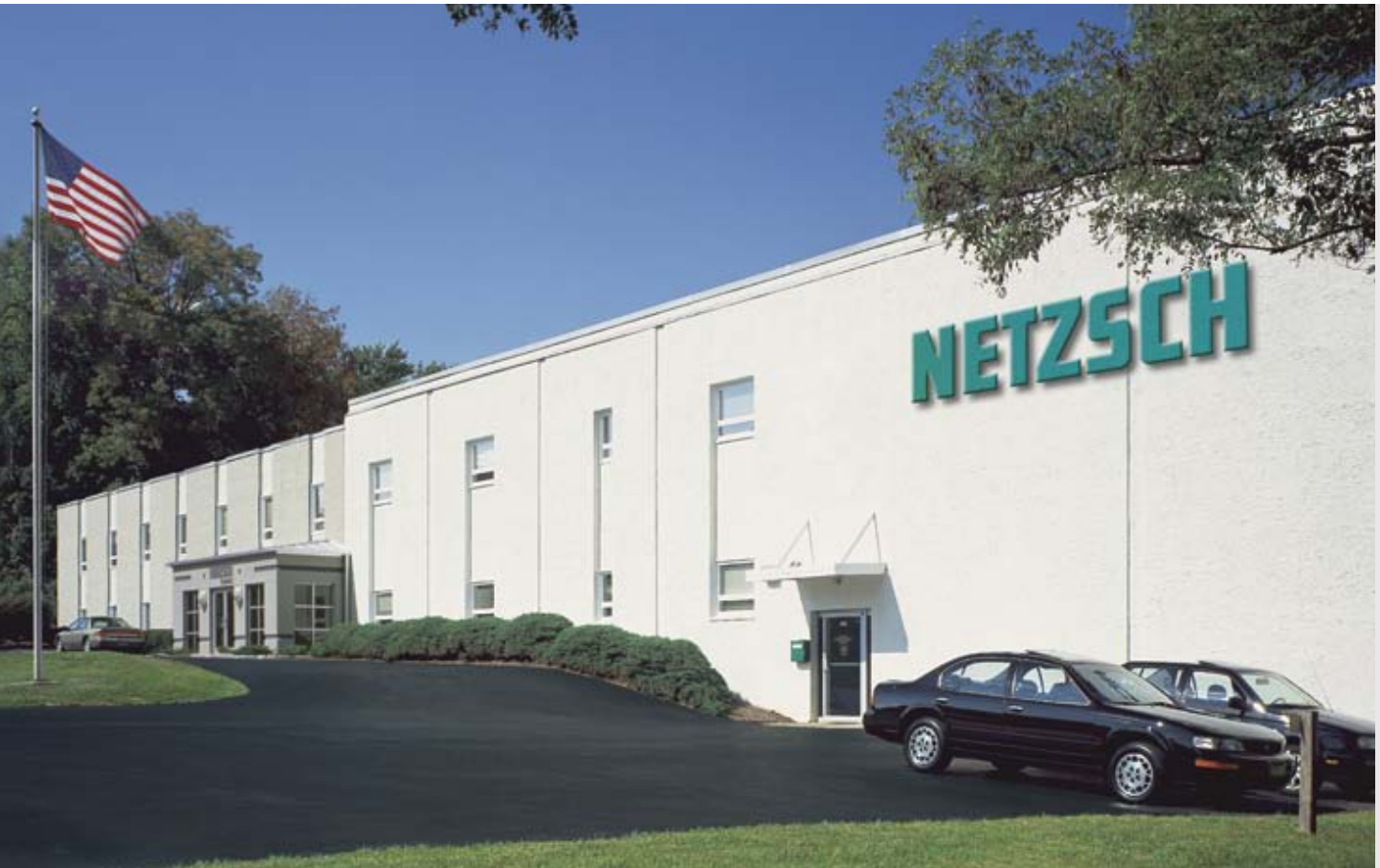
Exton, PA Facility
